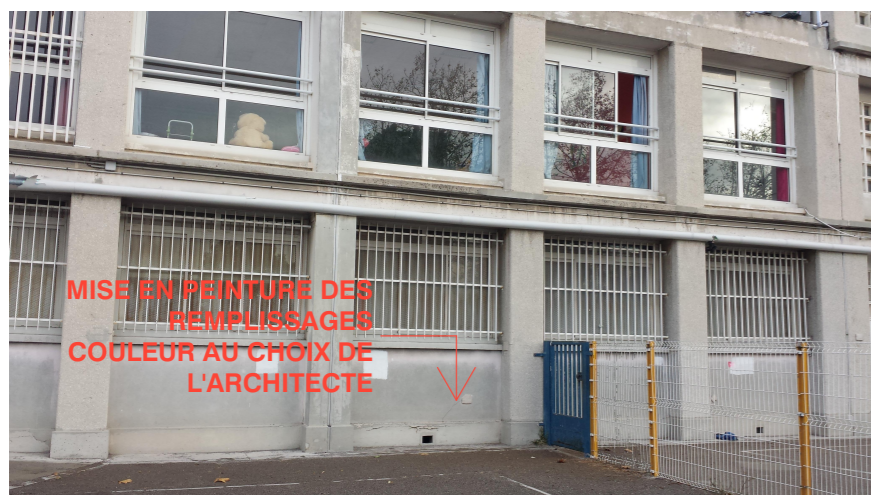
FACADE ECOLE MATERNELLE / REFECTOIRE - COTE COUR
