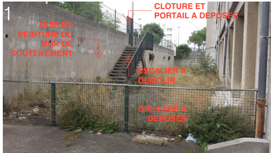
FACADE ECOLE ELEMENTAIRE - RUE DOURIANT "DOUVES"
