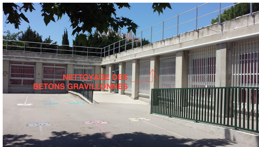
FACADE ECOLE MATERNELLE - COTE COUR
