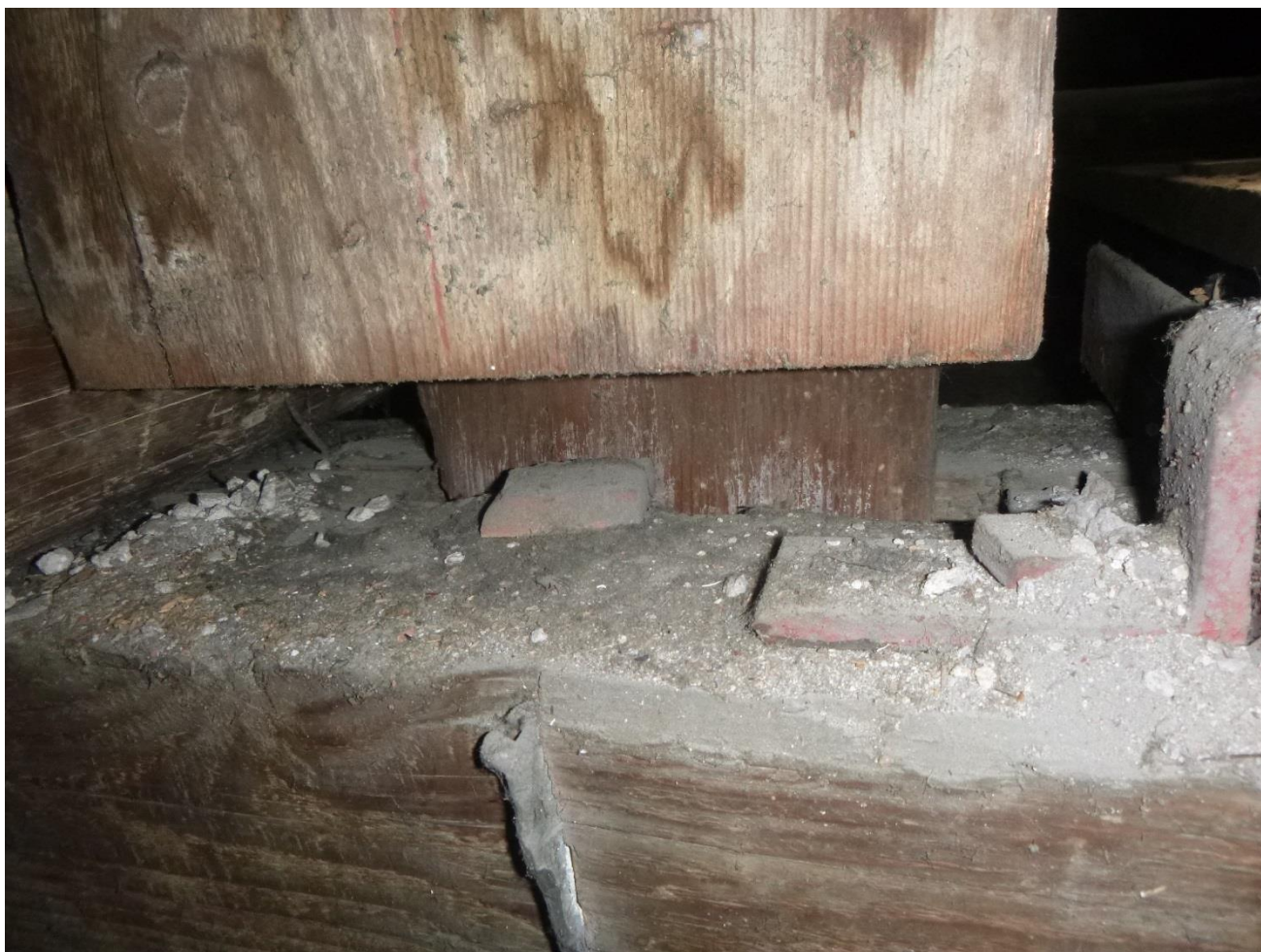
Photo 19 Assemblage poinçon/entrait
